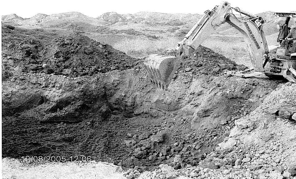
PHOTO 2 – Excavating diesel affected soil at Sterling 2-10.
