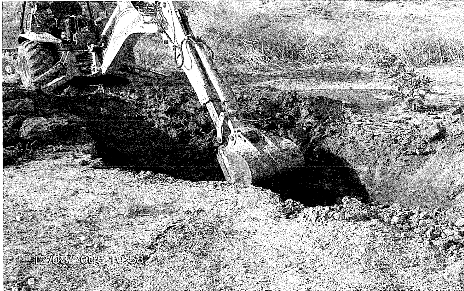
PHOTO 1 – Excavating sump at upper well pad (Sterling 2-10).
