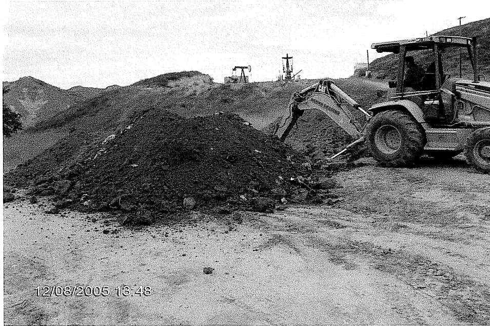
PHOTO 3 – Excavating trash fill with hydrocarbons at lower well pad (Sterling 1-10).
